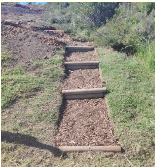
Block five new steps and pathway.
