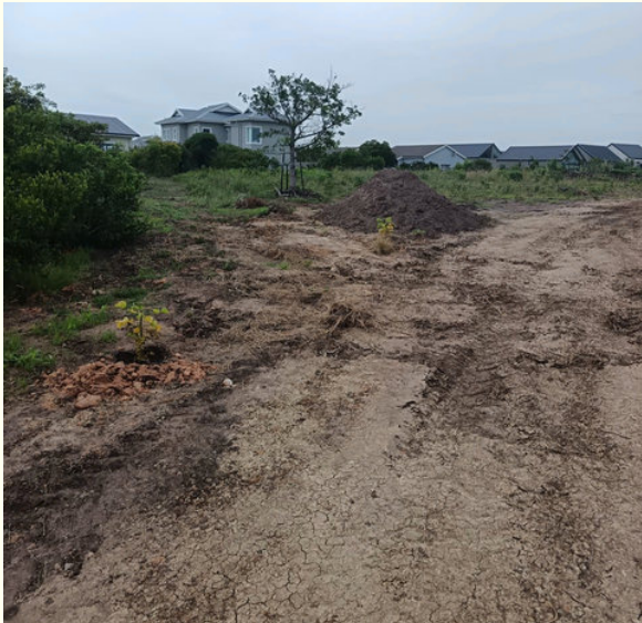
Laying of fresh topsoil in bock five.
